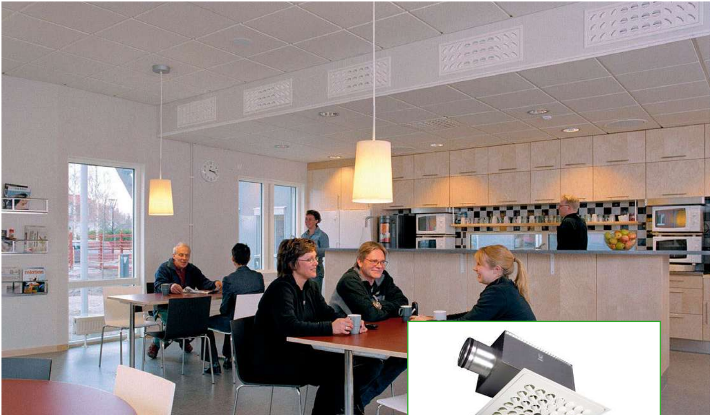
Swegon's disc diffusers have fully adjustable diffusion pattern that won't affect the pressure or increase the level of flow-generated sound. (Diffuser with commissioning box shown)
